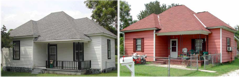
Note how changes in materials and architectural elements can alter the architectural integrity of a historic building. Integrity affects the architectural character of these buildings
