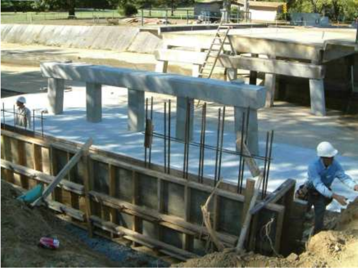
Figure 2-3: Widening of the Lily Flagg Bridge, October 16, 2003.
