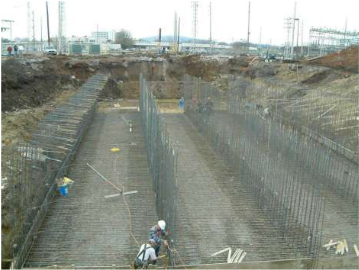
Figure 2-4: New Fagan Creek culvert under construction, December 12, 2003
